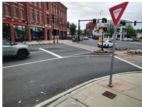
Image 8: Yield sign located in advance of crosswalk and intersection point.
