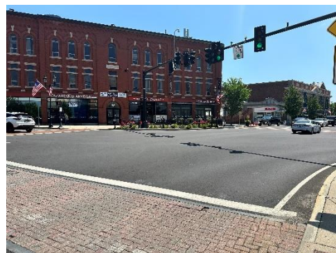
Image 6: Left-turn signal indications along mast arm over center of intersection.
