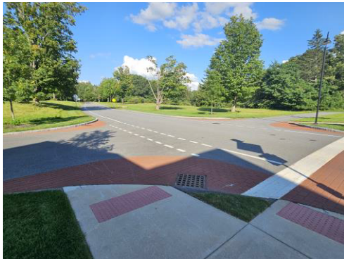
Painted Curb Extension, Devins, MA
