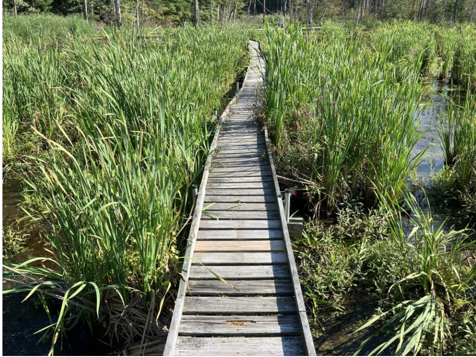
Replaced and damaged decking on the four-foot-wide boardwalk
